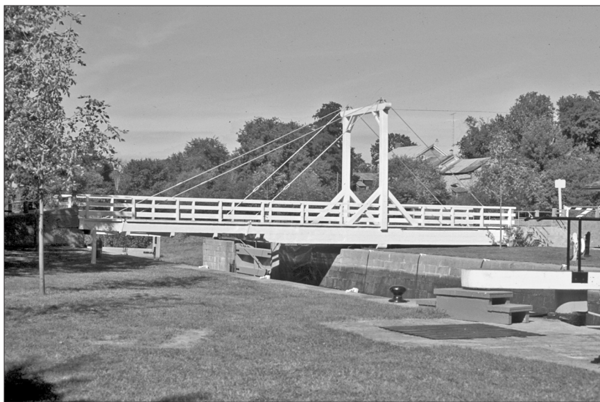
Figure 12. Upper Nicholson's timber swing bridge, as reconstructed in 1971. (Photo by author, July 1974)
