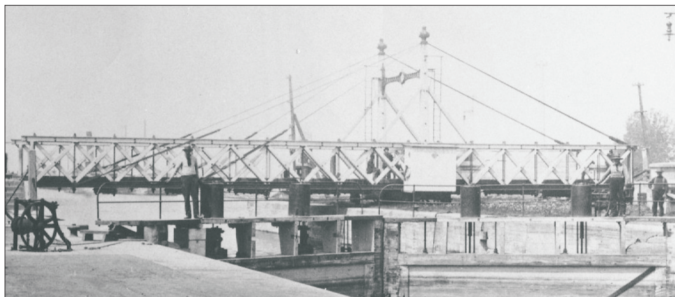
Figure 6. Lachine Canal Timber Swing Bridge, showing the evolved form of the mid-19th century Howe pony truss type of centre-bearing swing bridge designed by the Department of Public Works. (Library & Archives Canada, "Bridge at Lachine above Lock No. 5," C-081815, June 1903)
