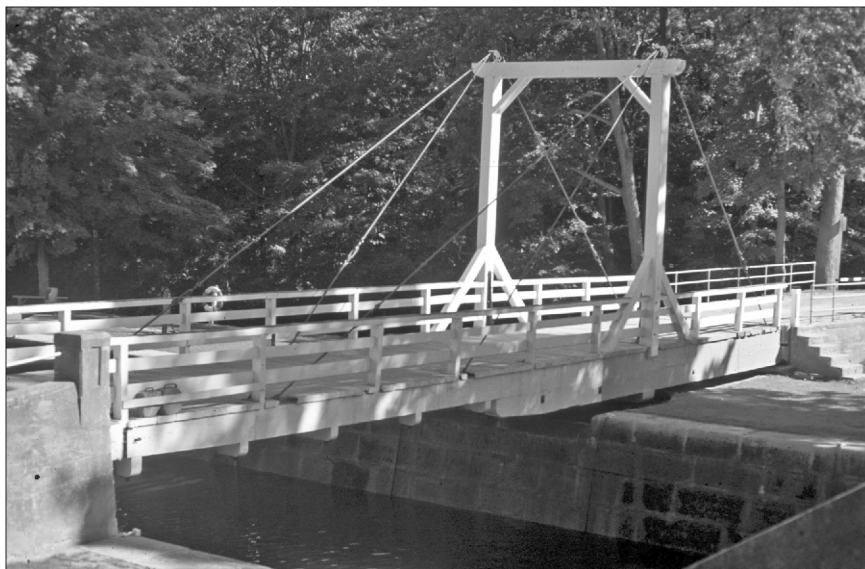
Figure 2. Jones' Falls Swing Bridge, a historic unequal arm, centre-bearing Rideau Canal type of timber swing bridge, reconstructed in 1960. (Photo by author, July 1974)
