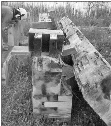
Figure 13. Double-tenon framing connections in evidence on the cut-up members of the Lower Brewer's swing bridge. (Eric Sunstrum, PWGSC, June 1984). The steel angles in evidence were added in 1981 to reinforce the interior joinery connections.
